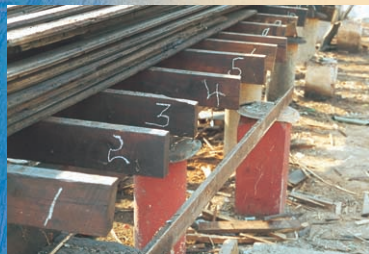
Dismantling the Wesleyan Methodist Church, 2000
