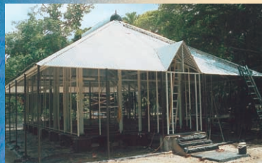
Completing the roof, 2000
