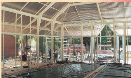
Re-erecting the Church in the Darwin Botanic Gardens, 2000
